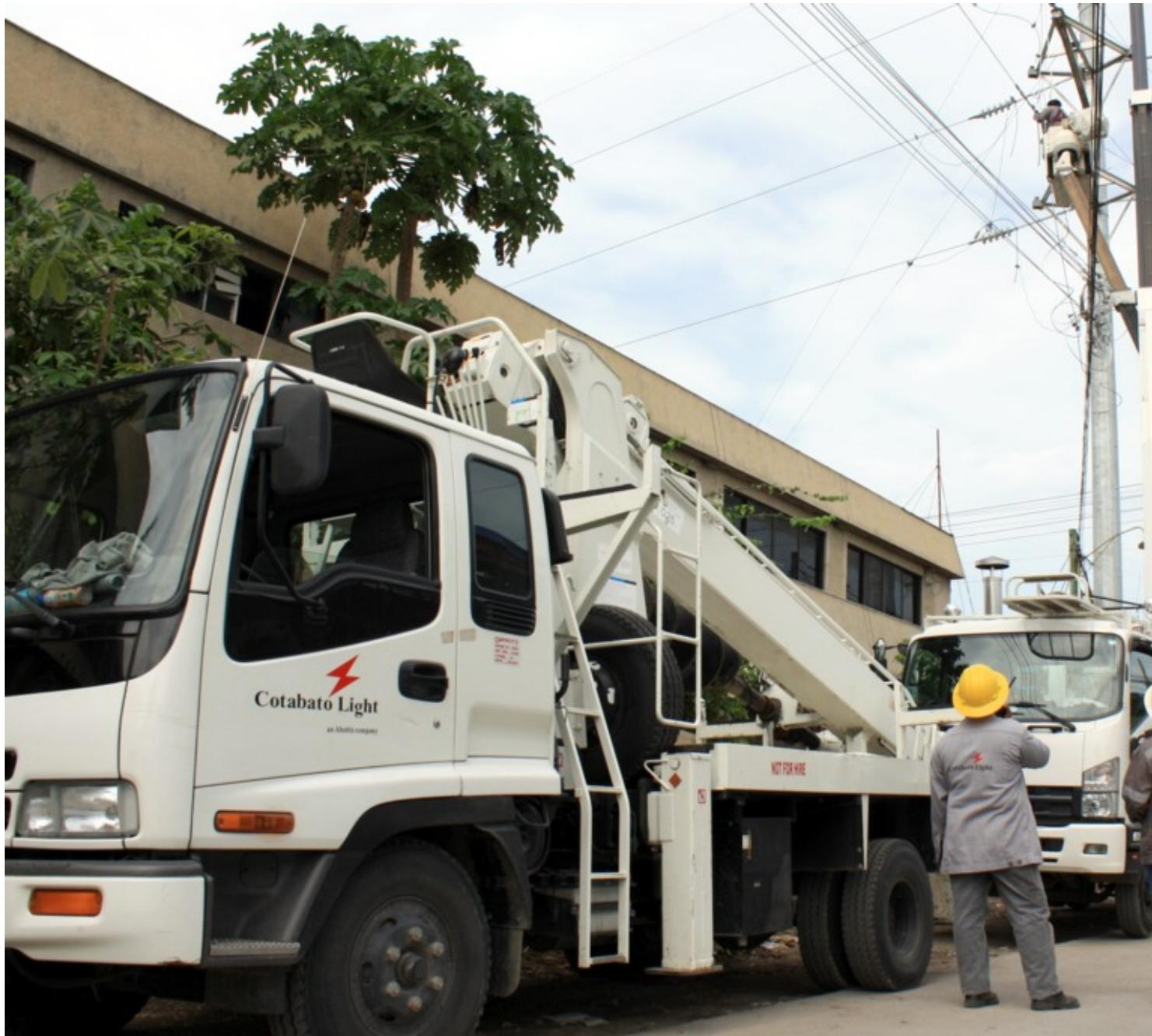
**TEAM AT WORK:** AboitizPower distribution utilities (DU's) Cotabato Light and Davao Light teams work together to speed-up the line stringing of the new Malagapas substation, while other team does the pole relocations.
