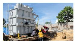
**SUBSTATION's POWER TRANSFORMER:** the Cotabato Light contractors are setting-up the hydraulic jacks to put the power transformer on its place.
